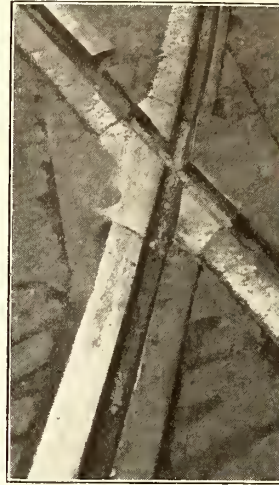
SPECIAL WORK ON CURVED TRACK REPAIRED
